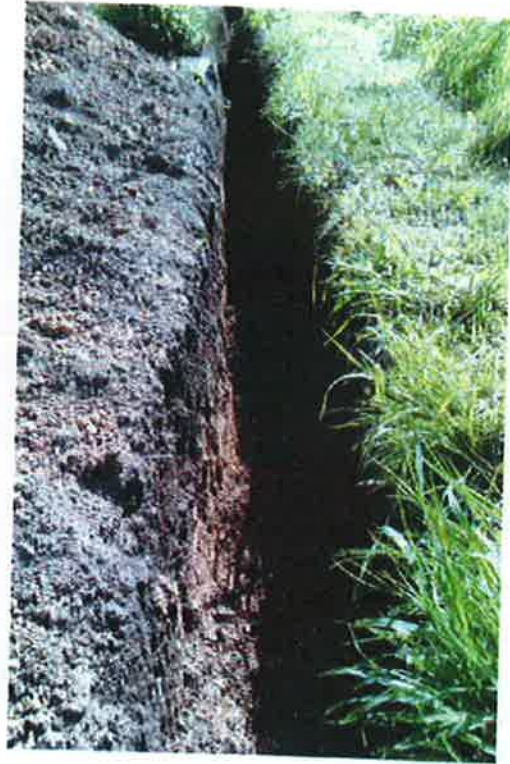
New trench for the water pipe.
